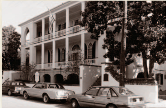
Old Marine Hospital (former Housing Authority Central Office)
